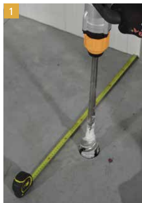
1 Measure and drill locations for anchor fixings.
