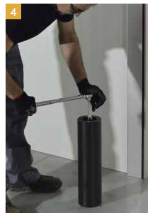
4 Locate anchor base and fix securely.
